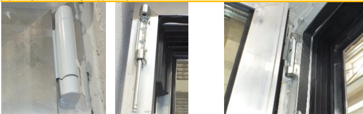
Opening-tilting window hinges type Unijet Mechanism
