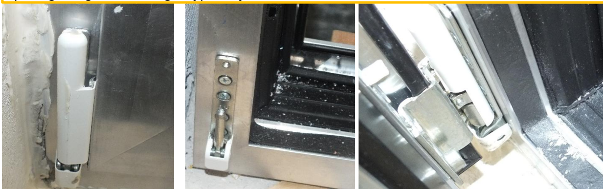
Opening-tilting window hinges type Unijet Mechanism
