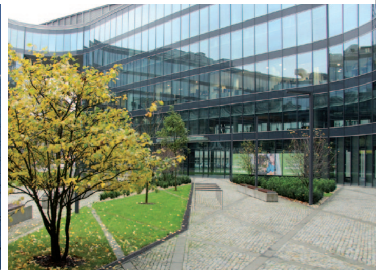
ČESKA REPUBLIKA OSTRAVA, NOVÁ KAROLINA PARK OSTRAVA - STRATOBEL STOPRAY 66.2 A STRATOBEL STOPRAY 66.2 - CMC ARCHITECTS - BREEAM VERY GOOD
